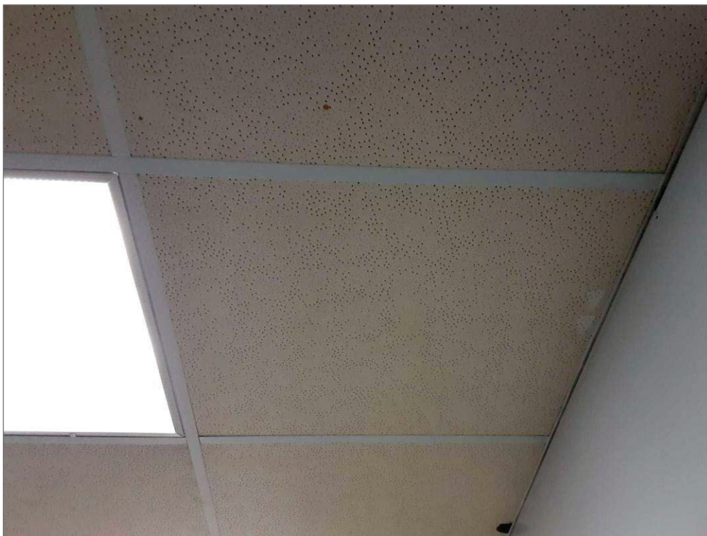
V9500 (Presumed Asbestos), 24x48 beige random pinhole, Ceiling, Ceiling Tiles (lay-in), Food Receiving Area (Location #: 80)
