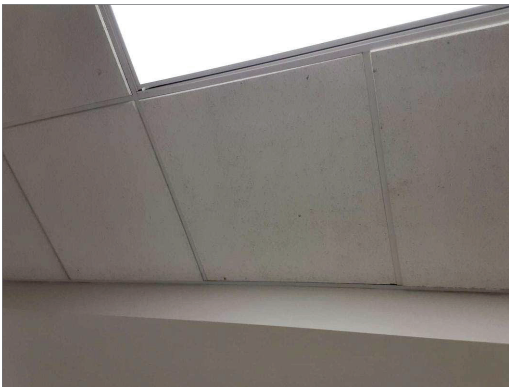
V9500 (Presumed Asbestos), 24x24 white rough textured, Ceiling, Ceiling Tiles (lay-in), Corridor 3 (Location #: 76)
