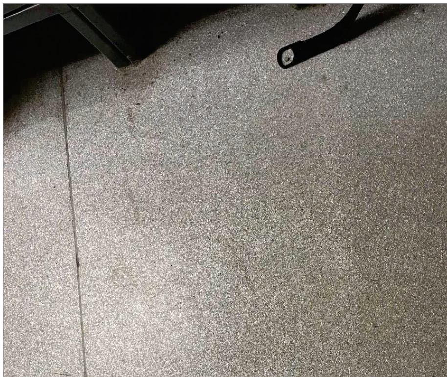
S0024A (Confirmed Asbestos), Grey, Floor, Levelling compound concealed by Vinyl Sheet Flooring, X Ray Control Room (Location #: 237)
