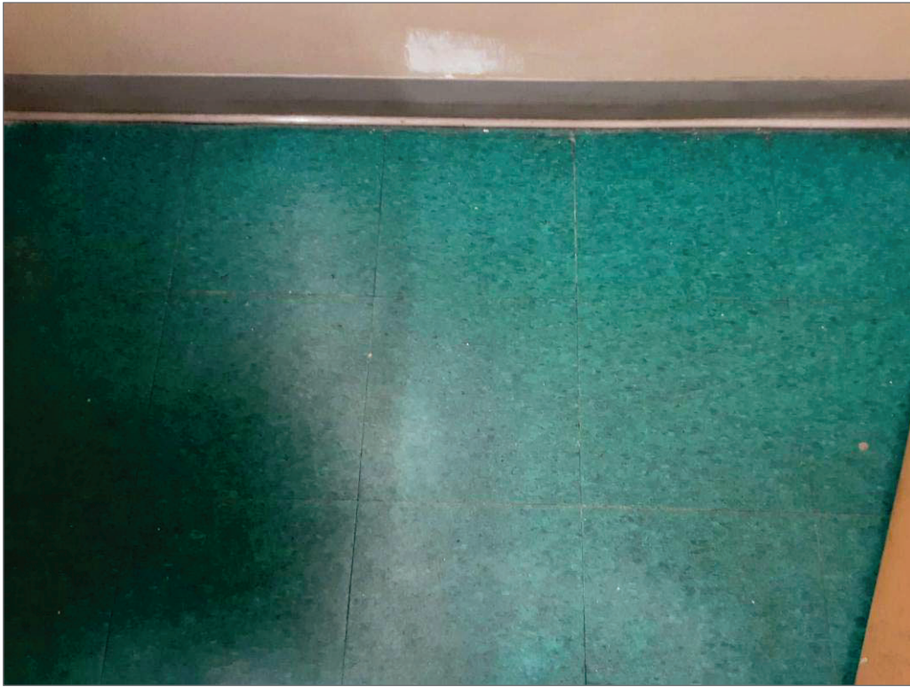
V9500 (Presumed Asbestos), 12x12 teal mottled, Floor, Vinyl Floor Tile, Universal Washroom (Location #: 247)
