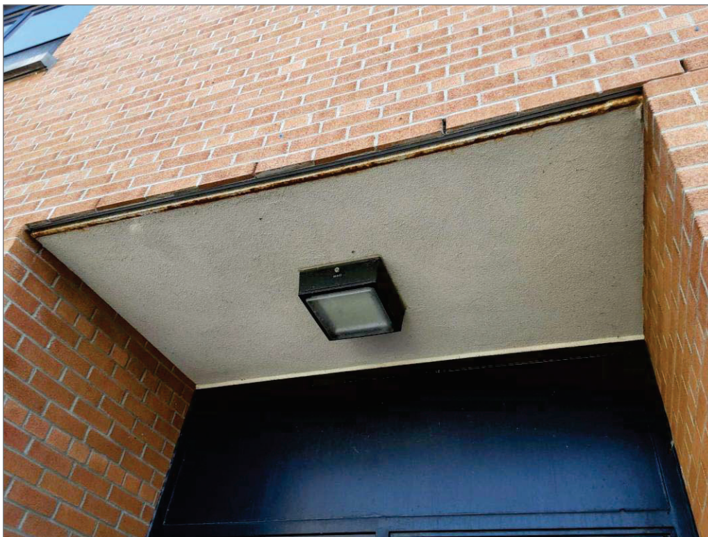
V9500 (Presumed Asbestos), Structure, Canopy, Texture Coat, Exterior (Location #: 403)
